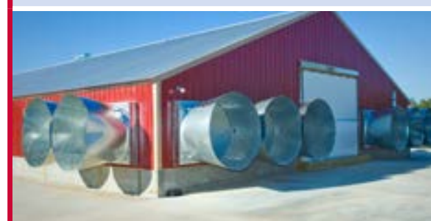
Figure 6.17 Example of a typical tunnel-ventilated house.
